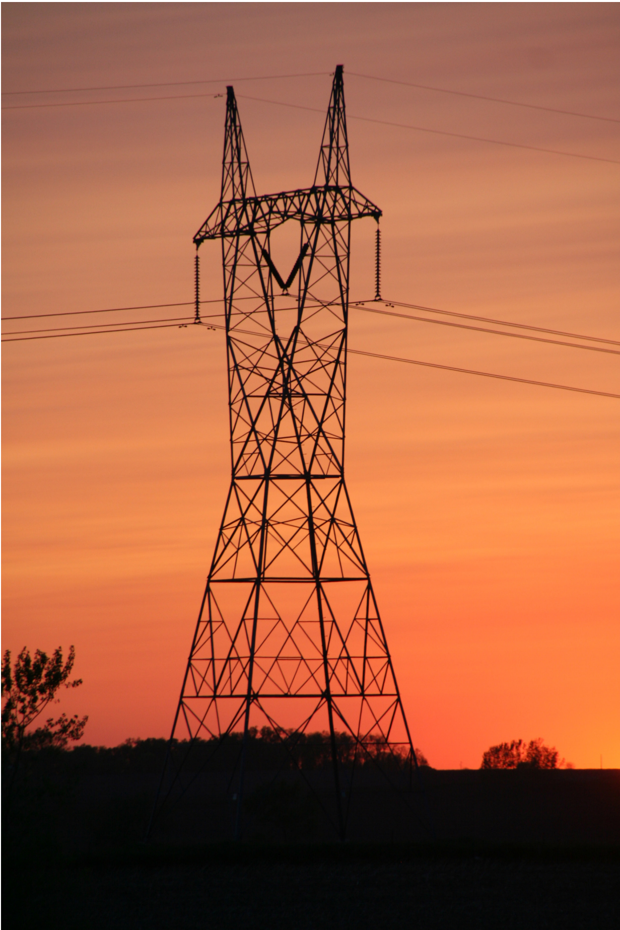
Transmission Line exiting the Deer Creek Generating Station, Elkton South Dakota
